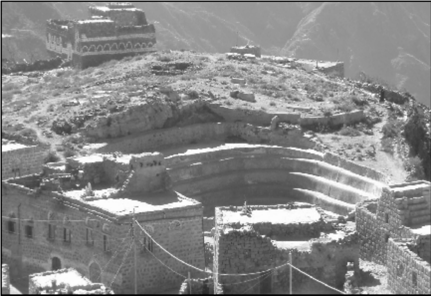
Figure 2: Public cistern on the escarpment of al-Jabin.
