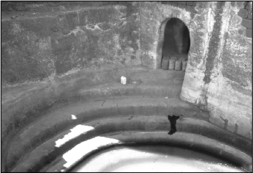
FIGURE 3: The Bayt al-Shaykh settlement's cistern.
